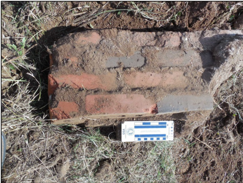
Figure 4.5: Feature 7, Segment of Long Brick Retaining Wall with Mortar
