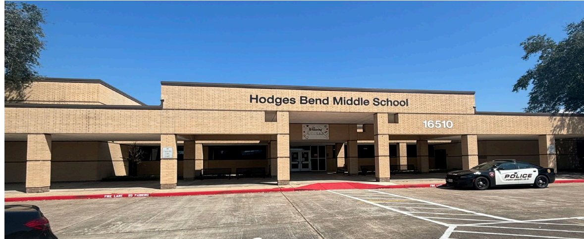
BP024 - Façade Upgrades & Renovations
