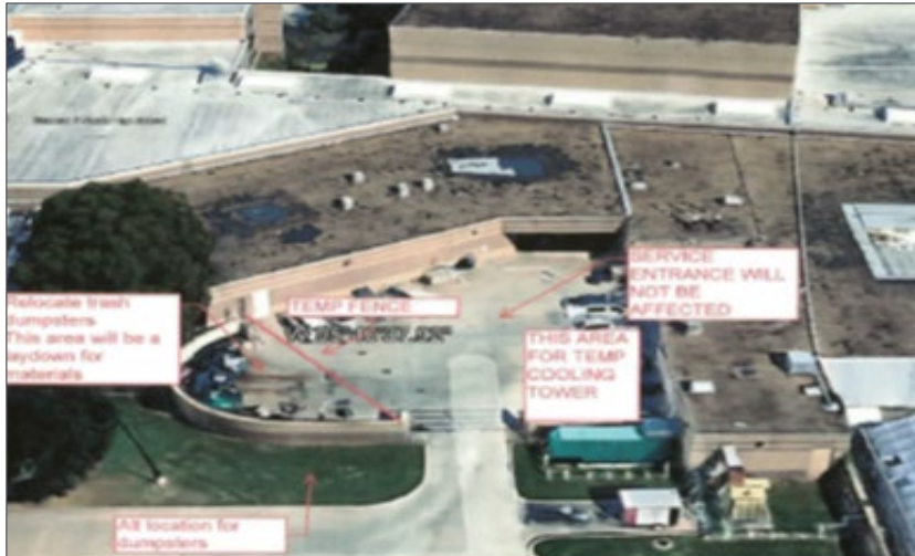
PKG046 – Austin HS Cooling Tower
