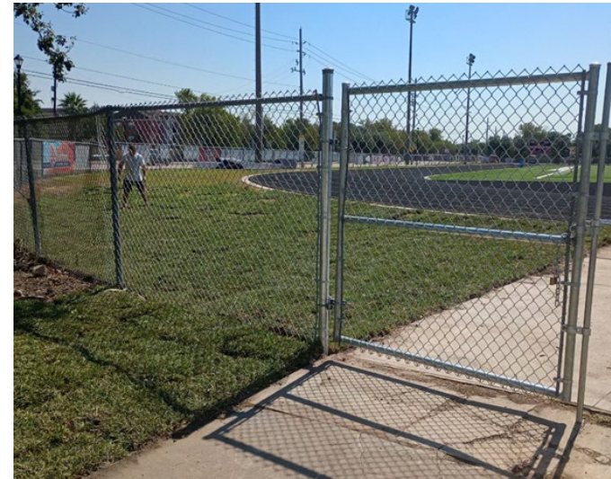
PKG056 – Fencing Upgrades
