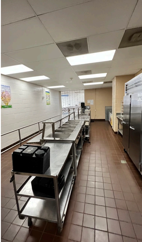
BP014 – Kitchen Renovations
